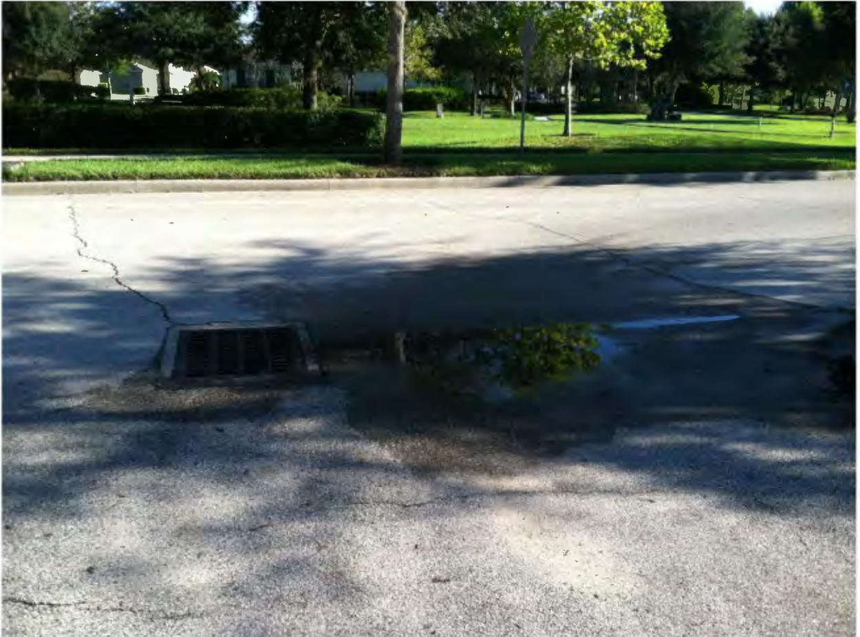
**60** Condition to be improved when resurfacing occurs. A temporary patch is recommended.
