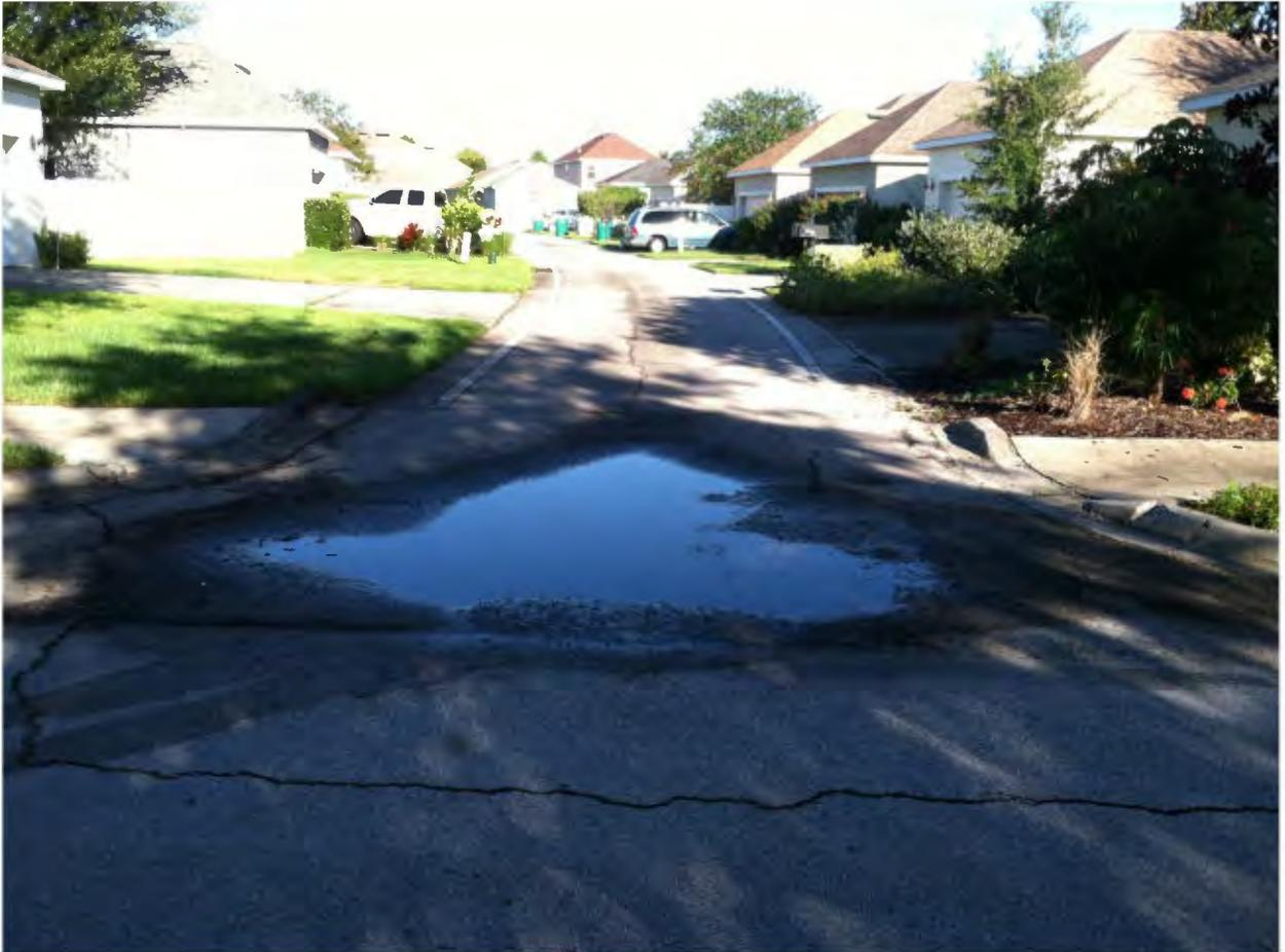
**47** This location requires that the existing asphalt and base be removed and replaced completely at the location where settling is occurring.
