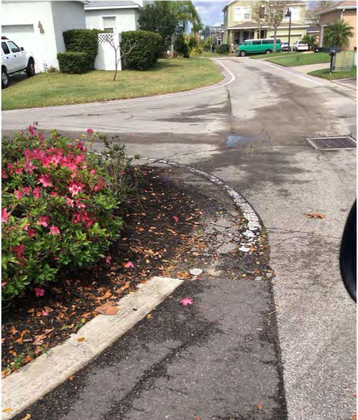
**64** This location which is partially within County ROW requires that the alley and roadway base be rebuilt around the inlet.
