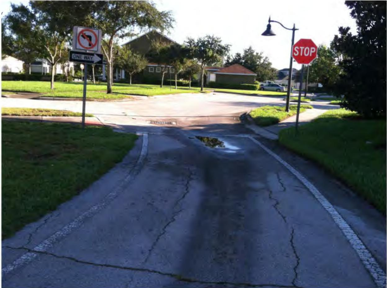
**49** Condition to be improved when resurfacing occurs. A temporary patch is recommended.
