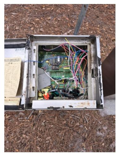
Controller (2) located on the right side of the main entrance appears to have been stollen. This proposal is to replace the controller and program the zones to operate as before
