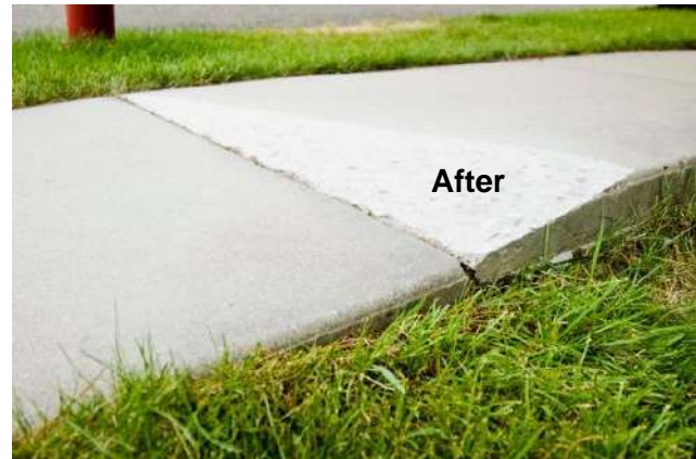
Figure 8: Precision Sidewalk Safety Work Example
