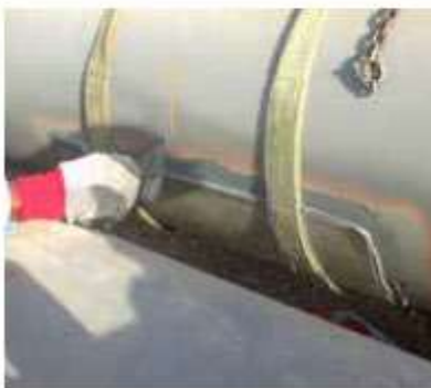
Bonding and shimming
