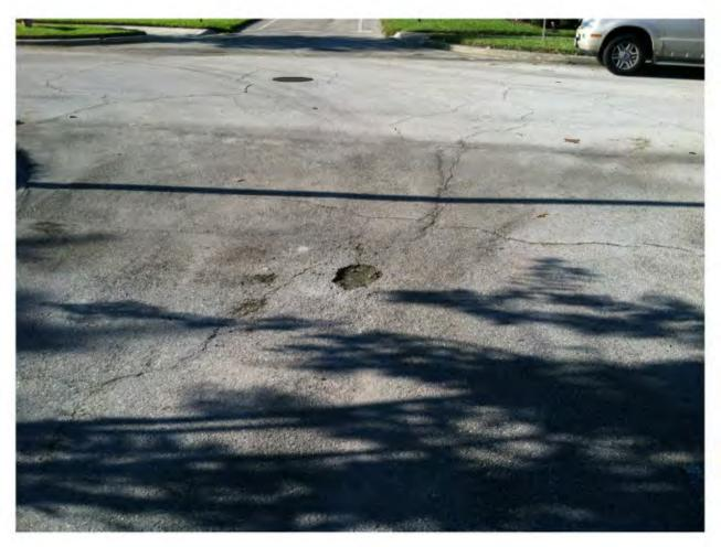
**50** This location requires that the existing asphalt and base be removed and replaced completely at the location where settling is occurring.
