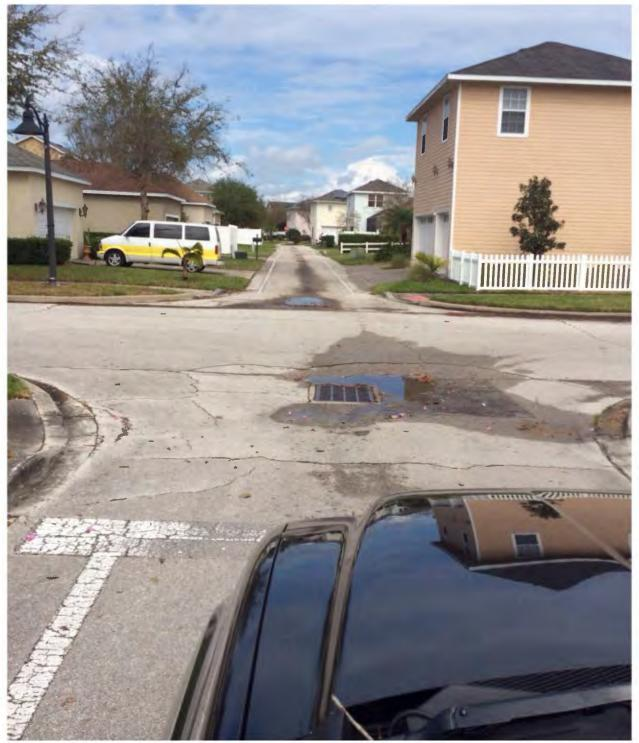
65 The radius at this alley intersection needs to be expanded to better accommodate truck traffic. This requires new base and pavement and should be completed with 2014 improvements. (Photo of this location taken from a Google Earth Image)
