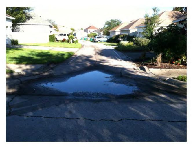
This location requires that the existing asphalt and base be removed and replaced completely at the location where settling is occurring.
